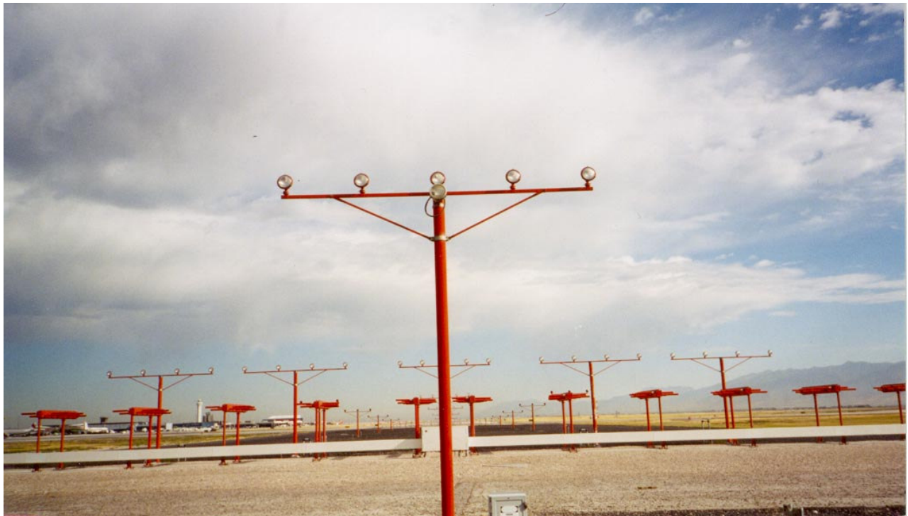
Figure 4-3. Approach lighting towers — fibreglass tubular poles
