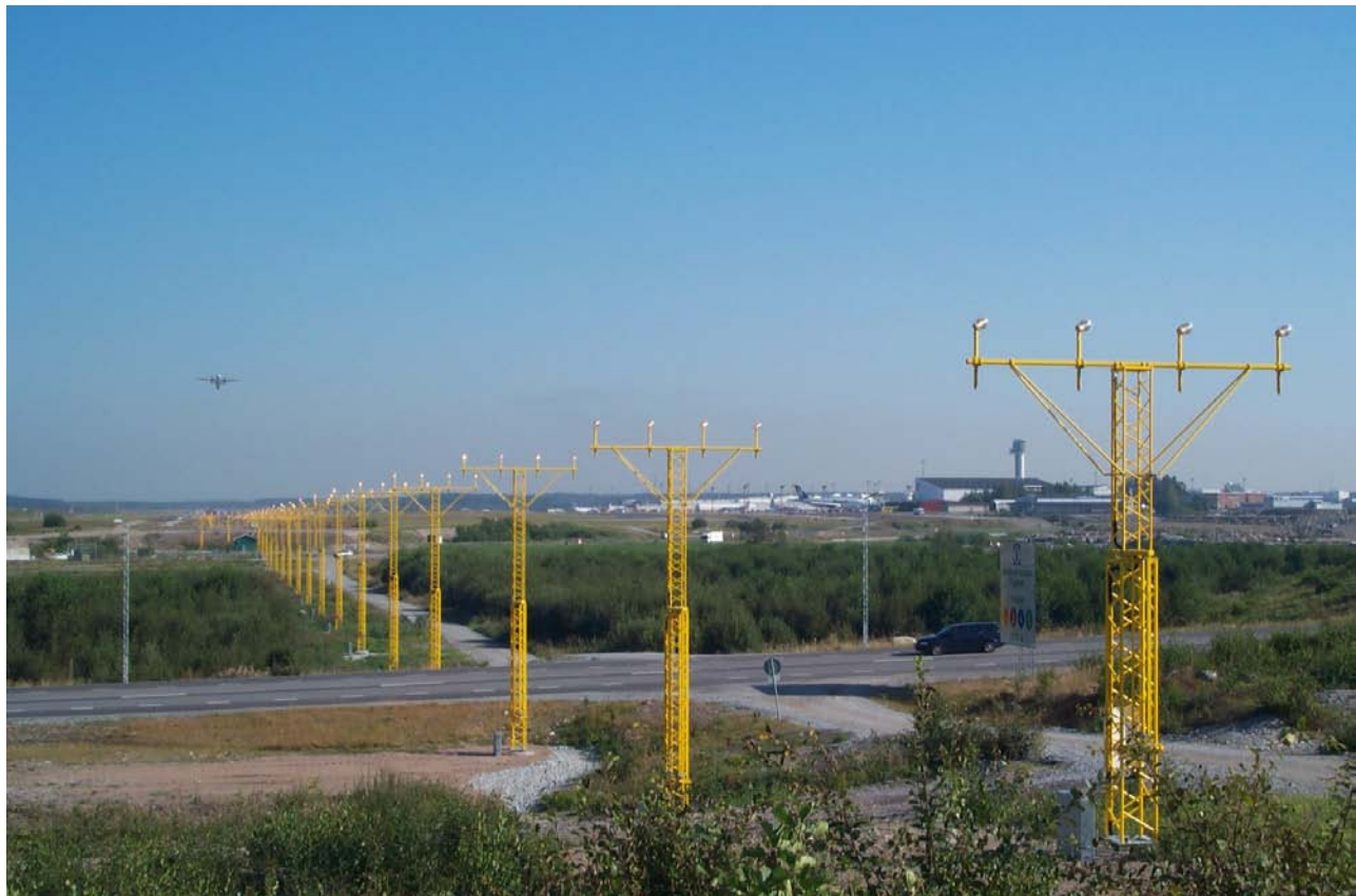
Figure 4-2. Approach lighting towers — fibreglass lattice structures
