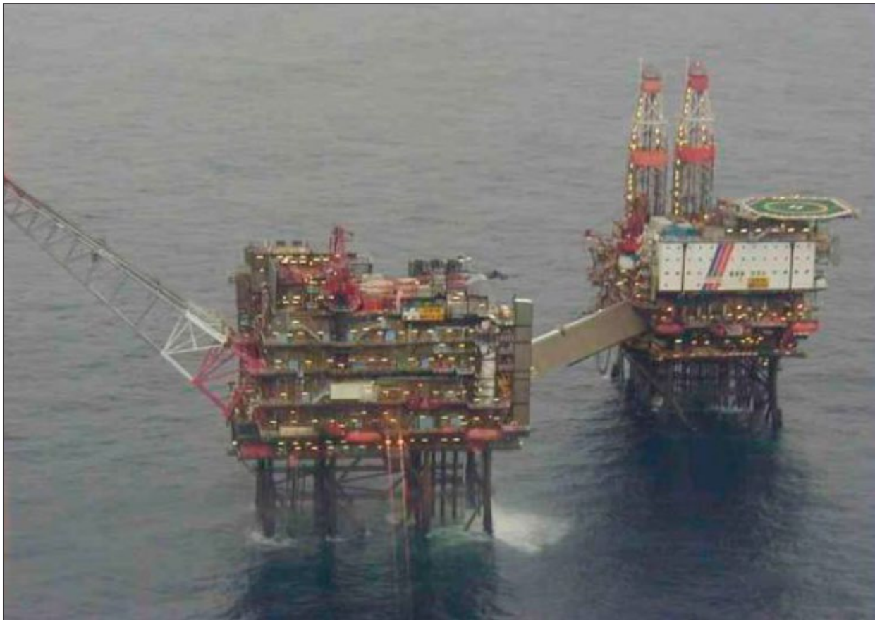
Figure I-1-1. A fixed platform with helideck above accommodation, bridge linked to a production platform
